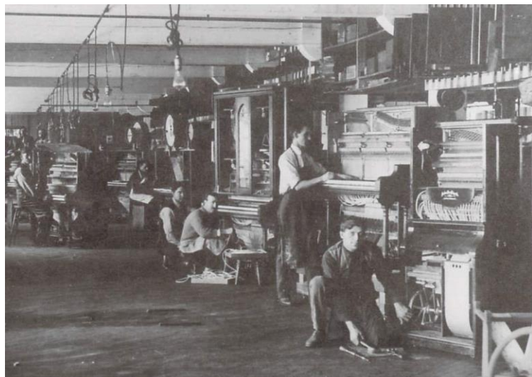
Fig. 11: Peerless final assembly area. Machines right to left: Peerless Style 44 with front removed, Peerless D, Peerless A orchestra, two early Peerless orchestras with exterior drums, some unidentified machines in the rear.
